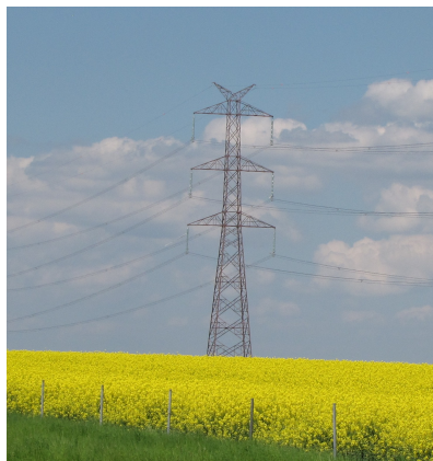
Figure 3.1: M3 transmission tower for a 400kV double track line [39]
