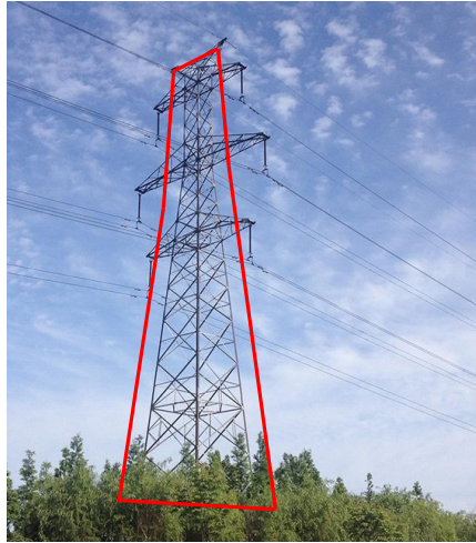
Figure 1.2: Body of a steel lattice tower
