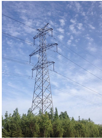
Figure 1.1: Steel lattice tower [40]
