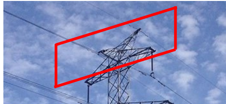
Figure 1.4: Body of a steel lattice tower
