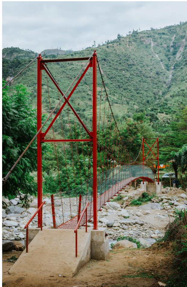
Fig 2 – Suspension footbridge
