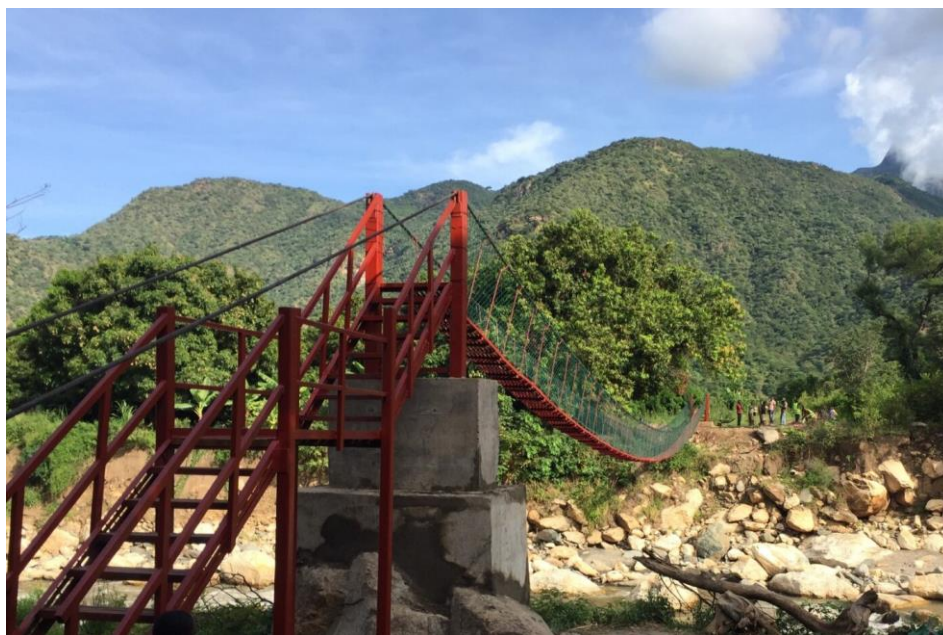
Fig 1 – Suspended footbridge
