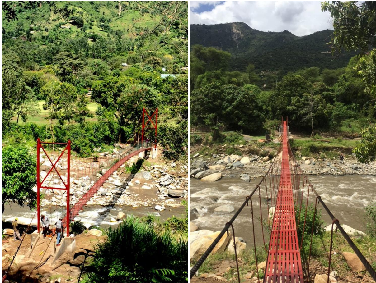
Fig 17 – Tamkal (left) and Sisit (right) footbridges
