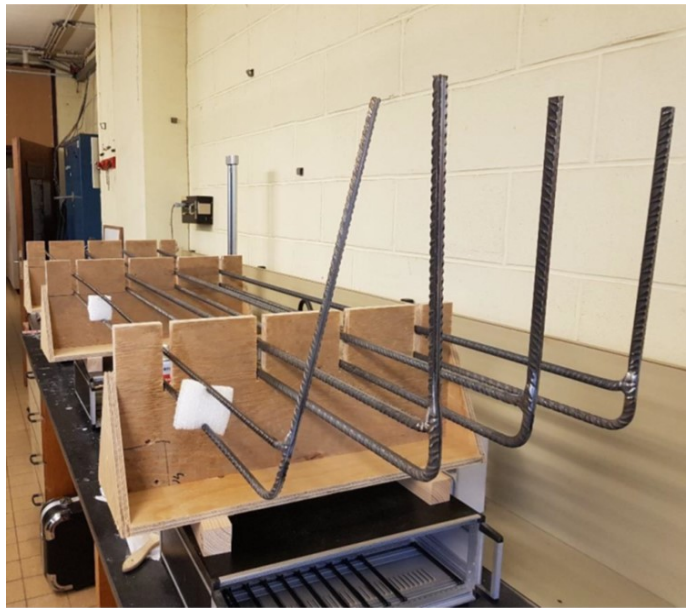
Fig. 4.16.: Reinforcement bars ready to receive the optical fiber
