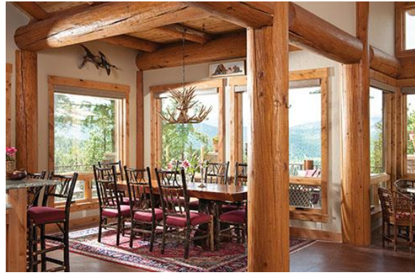
Figure 2 : Construction Poteau-Poutre [18] [19]
