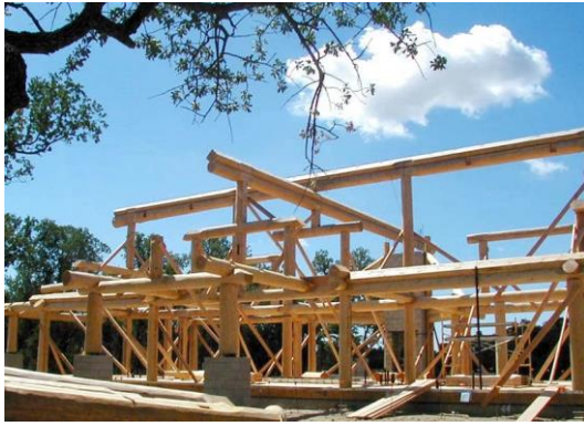
Figure 2 : Construction Poteau-Poutre [18] [19]
