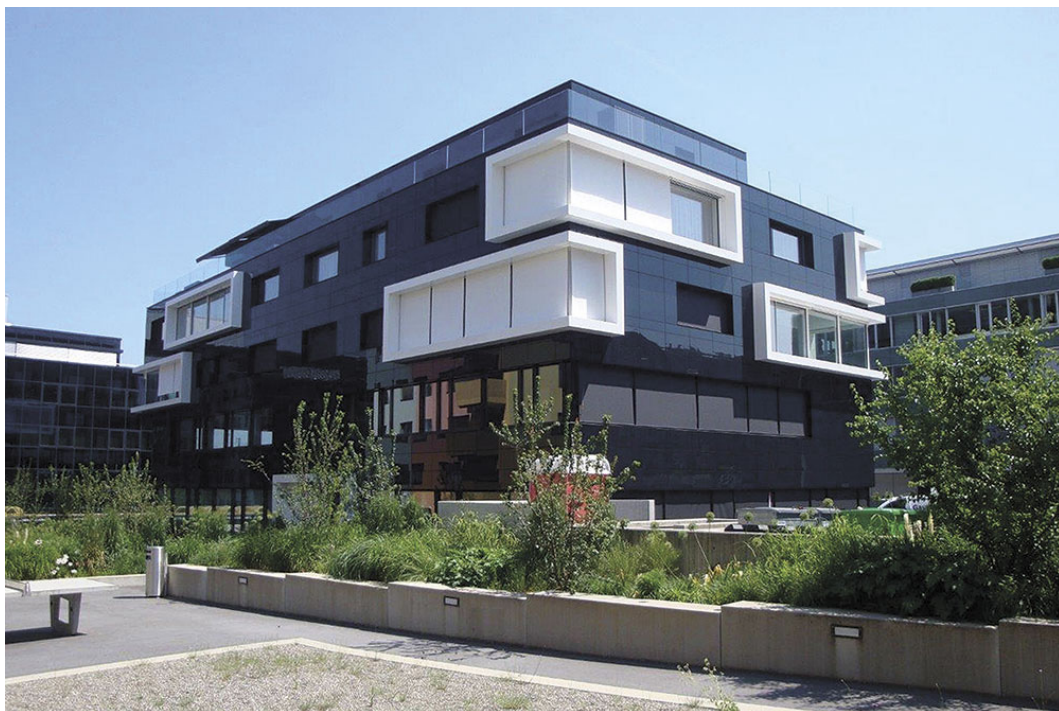
Figure 1.2: Application of building-integrated CIGS PV panels from [3].
