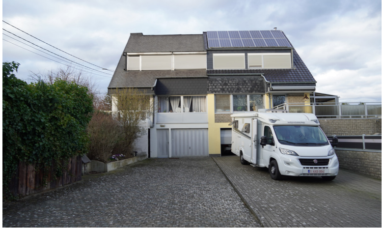
Figure 12: Semi-detached house in Kelmis
