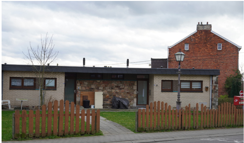
Figure 13: Semi-detached house in Kelmis
