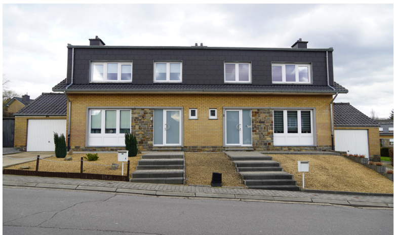
Figure 14: Semi-detached house in Kelmis
