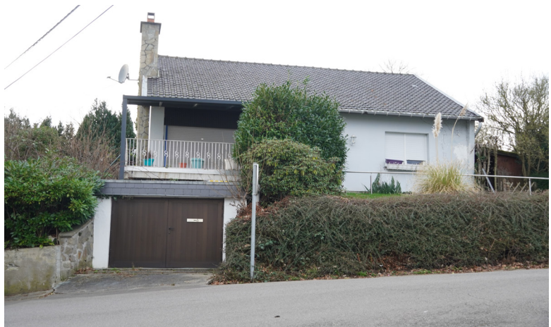
Figure 11: Single-family house in Kelmis
