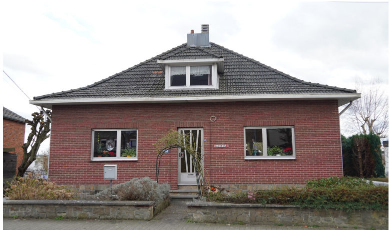
Figure 10: Single-family house in Kelmis
