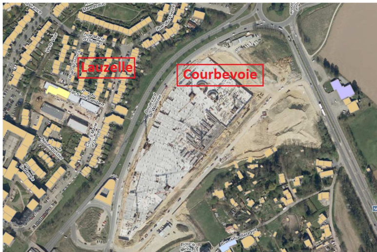
Figure 2.1.3 Works in progress for the construction of the new district (GeoPortailWallonia).
