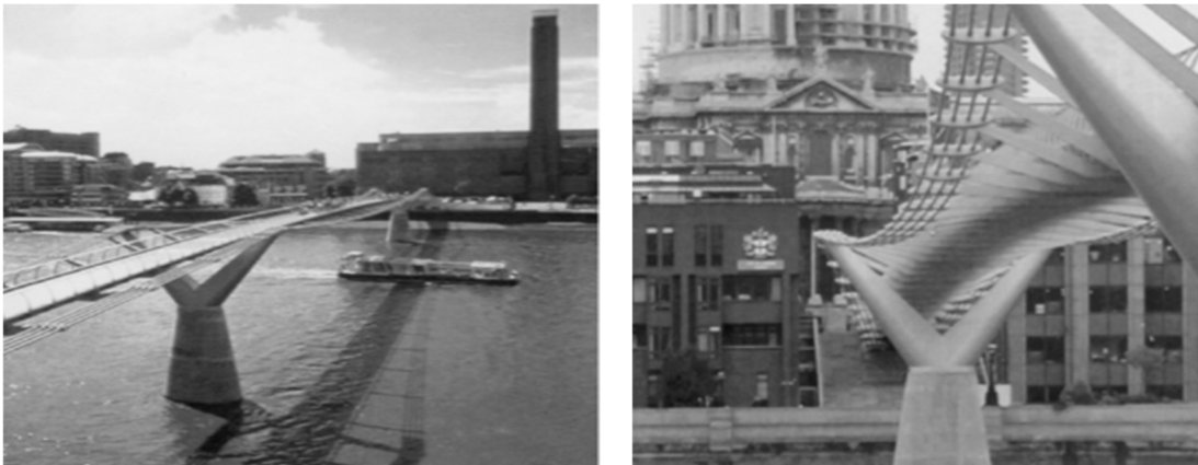
Figure 1.1.1 Views of the Millennium Bridge, London [36].
