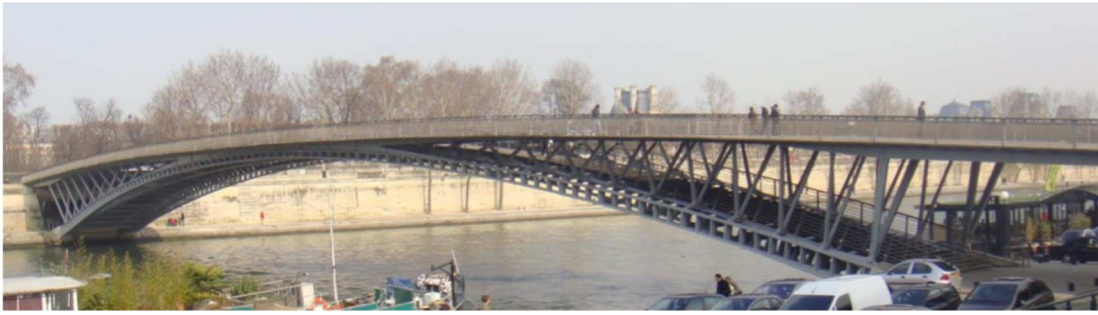
Figure 1.1.2 The Solferino Footbridge, today Passerelle Léopold-Sédar-Senghor, Paris.
