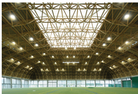
(a) Muroto Indoor Stadium
