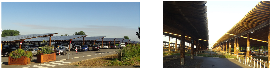
FIGURE 1.4 – Parking photovoltaïque de Pairi Daiza [15]
