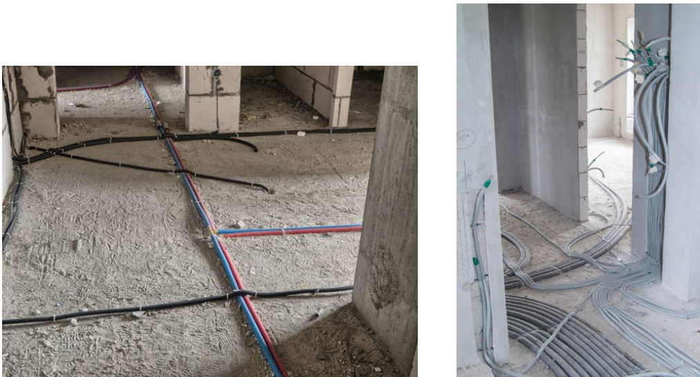
Figure 2: Construction sites with wires installed
