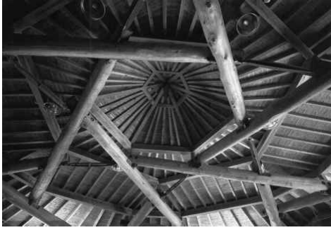
Figure 2.18: Charpente du Stonemason Museum (Photo: Kelkaku-Inc.) [18]
