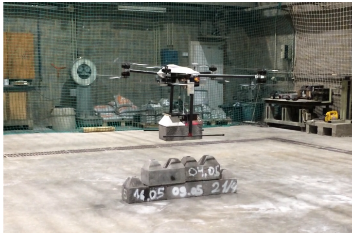
Figure 3.3: Drone building wall of dricks
