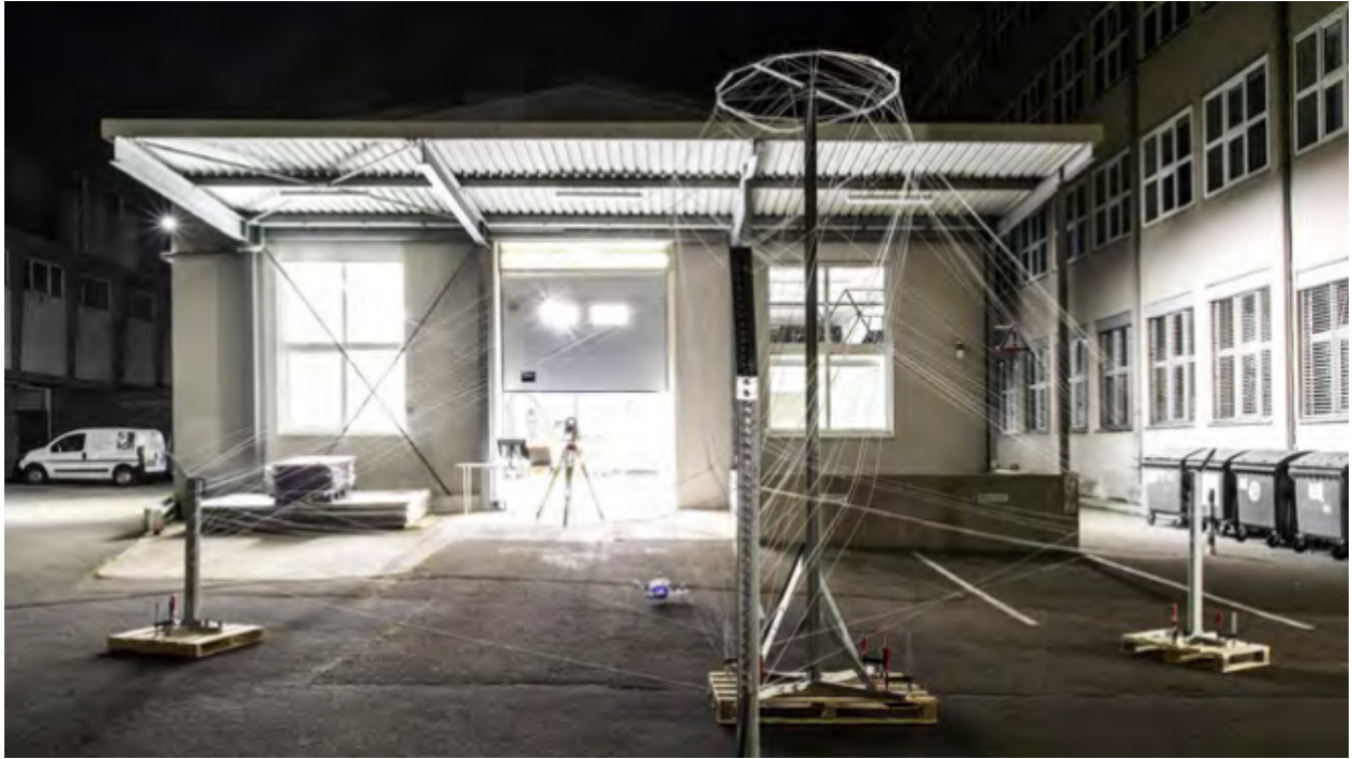
Figure 1.10: Fiber composite structure built by an UAV, guided by a system using a total station (Leica MS60) to position it spatially[9].
