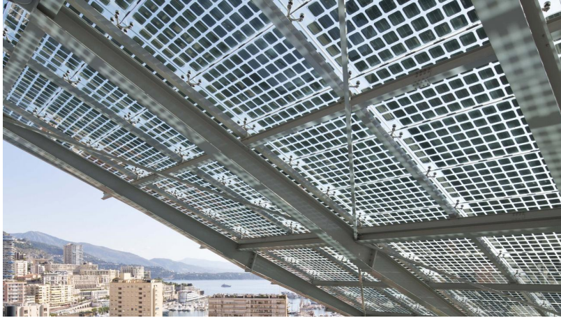
Figure 1.5: Example of flat glass including PV cells from [23]
