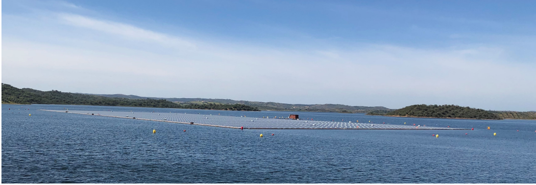
Figure 2.13: PV panel at the Alqueva dam in Portugal (Personal picture)
