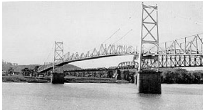
FIGURE 2.17 – Pont Silver Bridge en 1928 [27].
