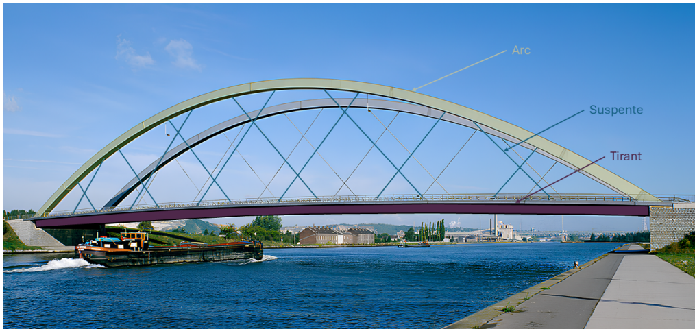
FIGURE 6.5 – Pont de Haccourt : structure de type bow-string.
