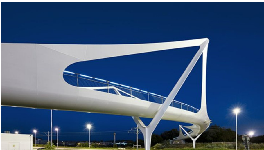
FIGURE 2.3 – Passerelle à Knokke, NEY & Partners (2007)
