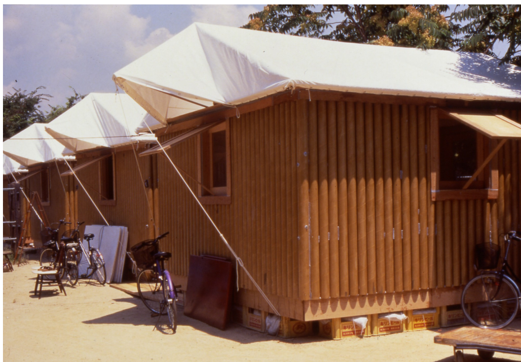
FIGURE 8.3 – Paper Log House, Shigeru Ban, Kobe (1995).
