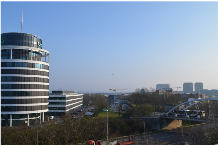
Fig 2: Photograph of the highway crossing of the Route d'Esch , 2024.
