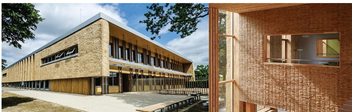
Figure 7. Use of straw on building façade and as interior finishing (Architype 2021, “University of East Anglia”)
