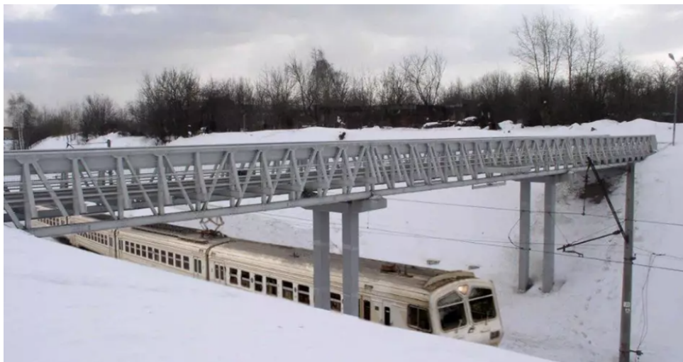
Figure 2.3: Concrete bridge reinforced with GFRP in Moscow, where deicing salt is abundantly used, to prevent corrosion[29]
