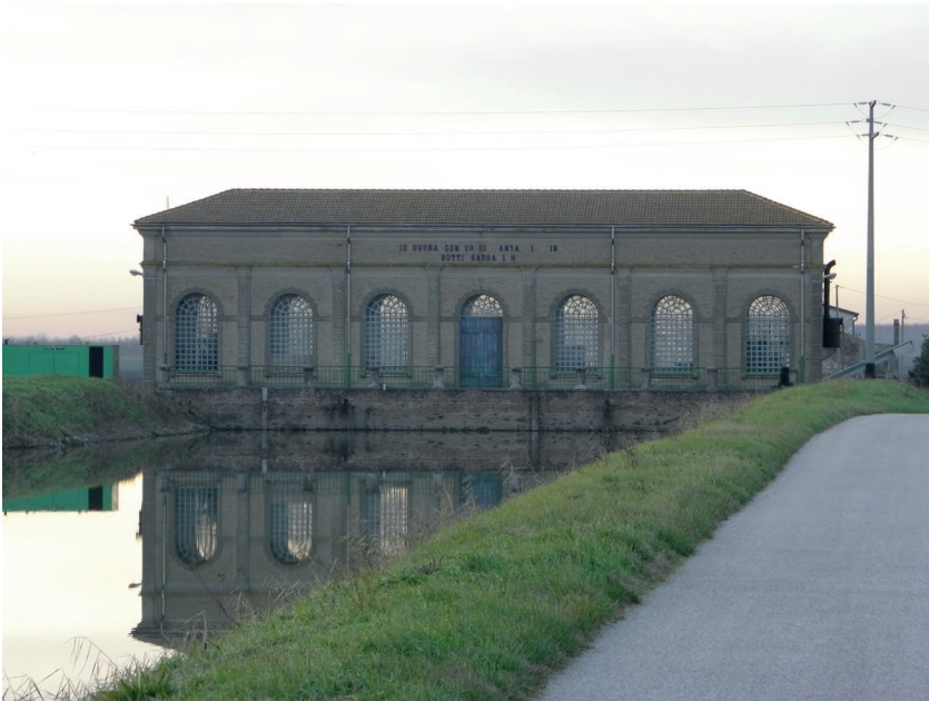
Fig.29 «Station de pompage Santa Giustina» (RAVENNA TODAY 2018)
