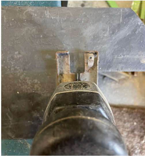
(a) Slate cutting
