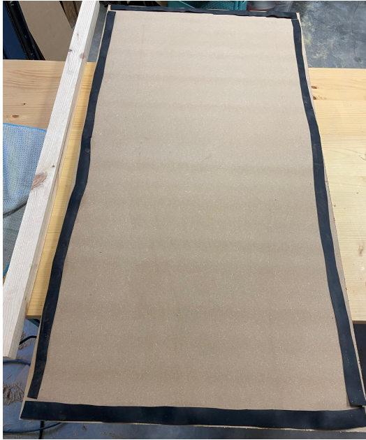
(a) Sealing of the base and frame
