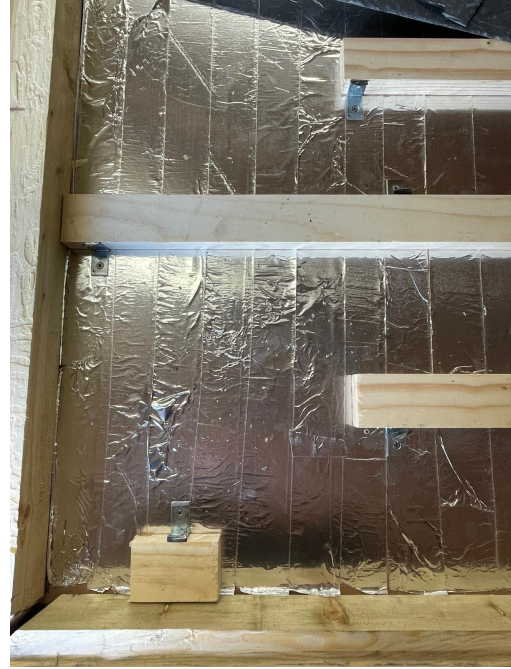
(b) Supports to hold the slates
