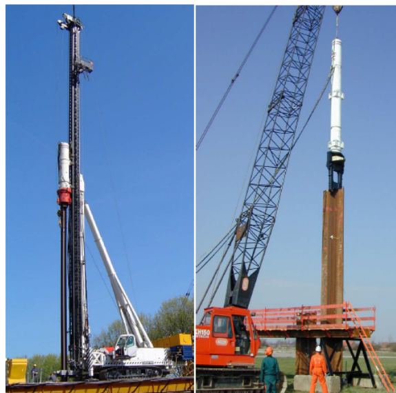
Figure 3.9: Pile driver and pile guide [13]
