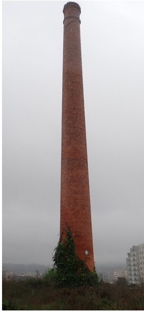
(a) Chimney without a base.
