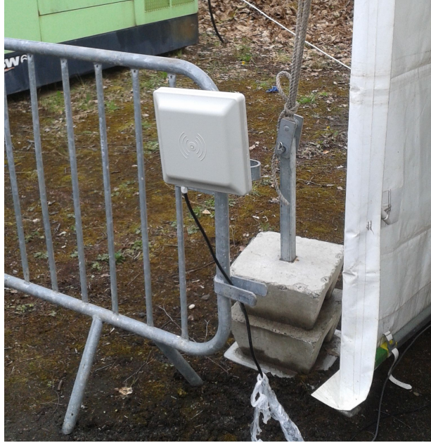
Figure 6.3: Installation of the antenna at the finish line
