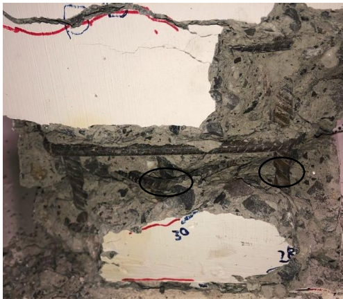
Figure 86 - Rupture des armatures colonne C2C
