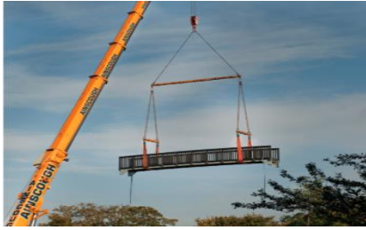
Figure 28 KLP recycled plastics footbridge near Rickmansworth in Hertfordshire (England) (ECS Engineering Services, 2014)
