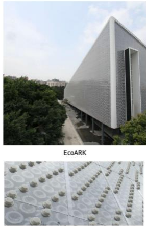
Figure 31 Polli-Bricks used to construct the Pavillion EcoARK in Taipei, Taiwan (2010) (MiniWiz, s.d.).
