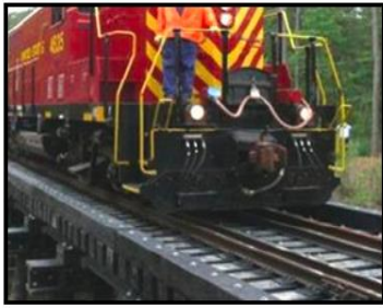
Figure 24 First railroad bridges made of almost 100% recycled plastics at Fort Eustis, Virginia (2010) (J. S. KIM, s.d.)
