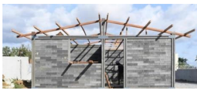
Figure 37 Classrooms in Côte d'Ivoire, Plastic blocks made by Conceptos Plásticos (Conceptos Plásticos, s.d.) (UNICEF, 2019)
