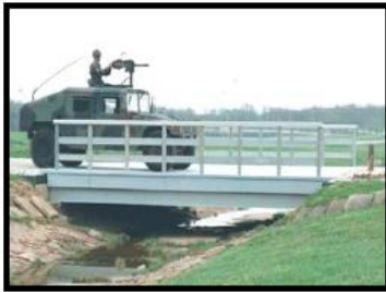
Figure 21 First vehicular bridge at Fort Leonard Wood, Missouri (1998) (J. S. KIM, s.d.)
