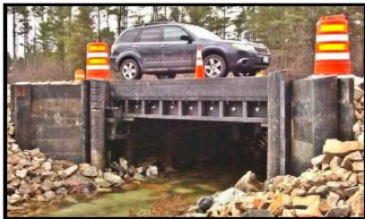
Figure 25 First highway thermoplastic bridge made of almost 100% of recycled plastics at York, Maine (2011) (J. S. KIM, s.d.)
