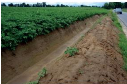
Photo 2. Fossé-talus. source : (SPW/EDIWALL, 2021)
