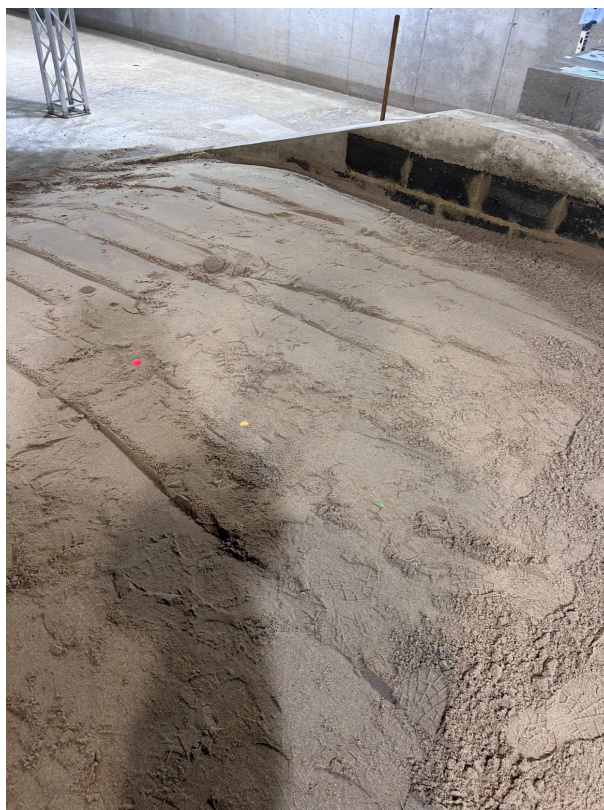
FIGURE 5.39 – Pose des balles
