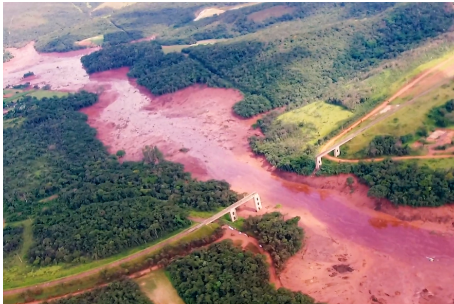
FIGURE 1.2 – Rupture du barrage de Brumadinho
