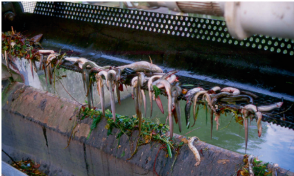
Figure 4: Eels collected from trash rack at Wahnhausen power station (Bruijs et al., 2009)
