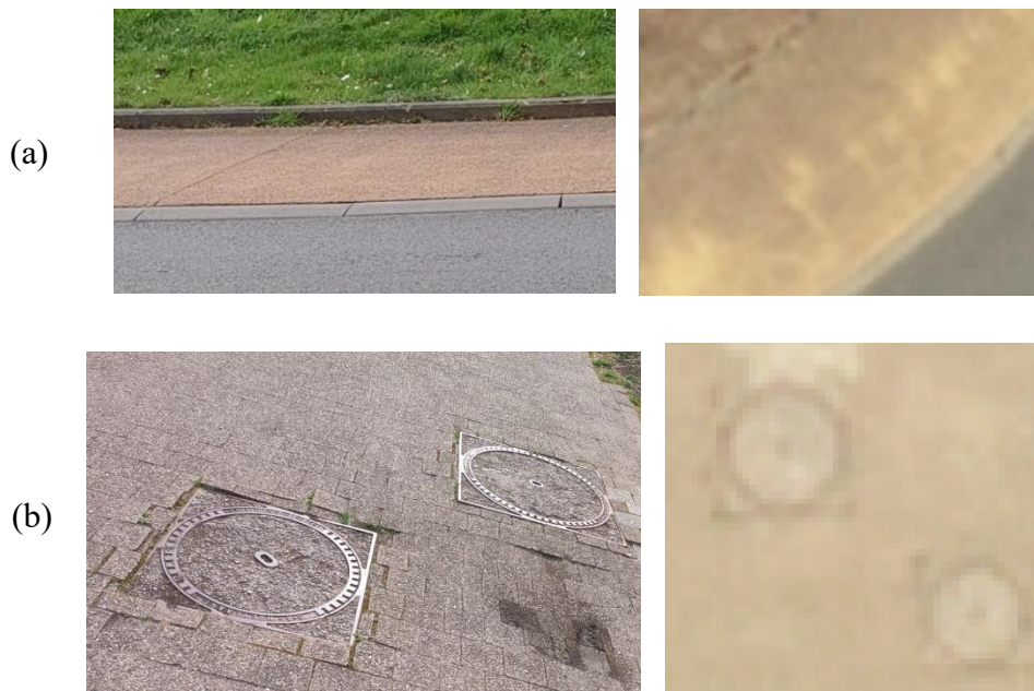
Figure 14. Field image and snapshot from orthophoto – (a) Concrete and (b) Concrete drain cap
