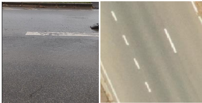
Figure 15. Field image and snapshot from orthophoto – Asphalt Roads
