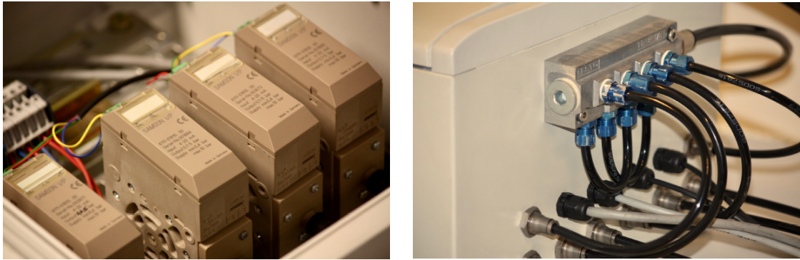
Figure 2.18: The I/P converters and the pressure distributor [4]
