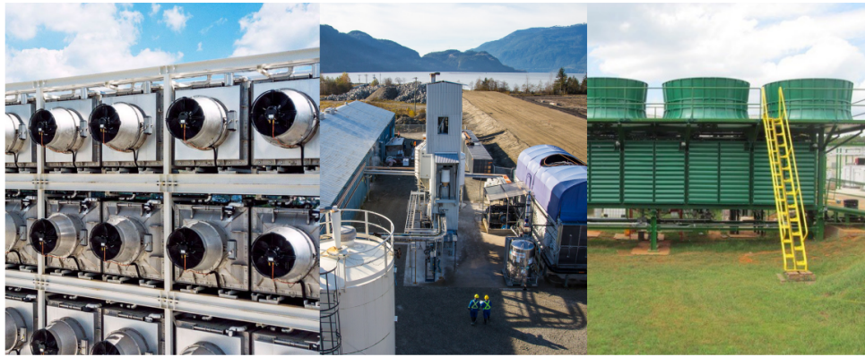
Figure 2.1: DAC plants from the three main companies. Starting from the left : Climeworks (Switzerland), Carbon Engineering (British Columbia) and Global Thermostat (Alabama). Figure taken from [14].
