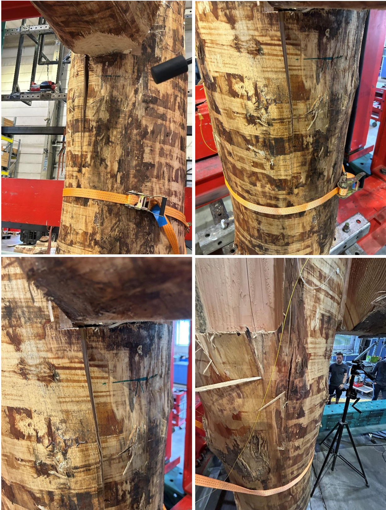
Figure 65: Views of the cracks observed on the column after the test. Source: Serena Van Nimwegen.
