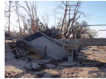
Figure 1.8: Jetty broken in Cardwell (Source: DSITIA).
