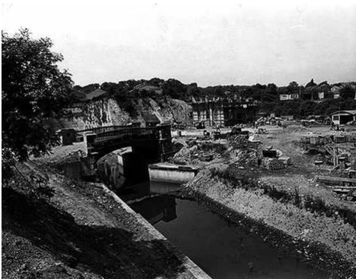
The construction in the late 1970s.
