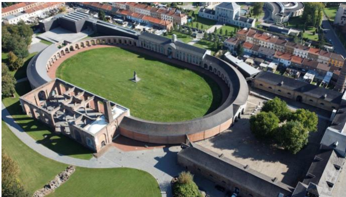
View of the site from above. (Source: MACS)
