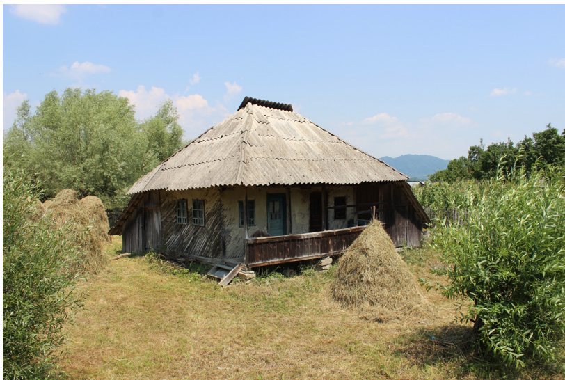
The vernacular culture of self building and the resulting extensions of the house (Source: by the author)
