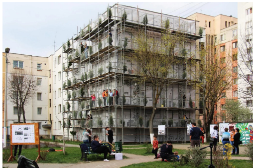
Improving Tudor- a research installation done during an international architecture and urbanism workshop, in search for ways to rehabilitate the socialist blocks of flats, both physically and morally (Source: Manopera.com)
