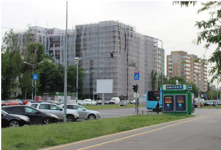
The Program of Thermal Rehabilitation put to work in the neighborhood of Drumul Taberei, creating the image of a veil covering the existing facade (Source: by the author)
