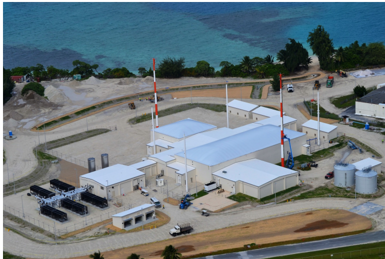
Figure 2.1: Space Fence Radar : the smaller off-white roof covers the emitting antennas while the larger one houses the receiving ones. The white poles help calibrate the radar. Image from [5]
