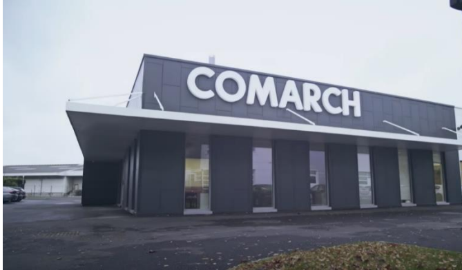
Photo 1: Comarch data centre building in Lille (Comarch France, 2018)
